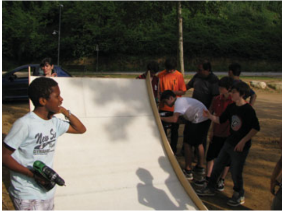
FIGURE 1. Building the skater park in Arbucies, 2001. (Photo by author)
